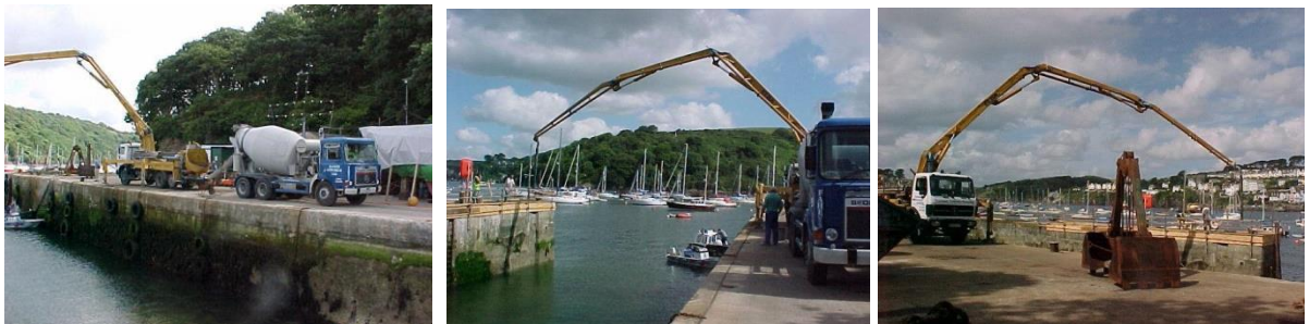
A long reach concrete pump was used to transfer concrete from lorries on the inner storage area
