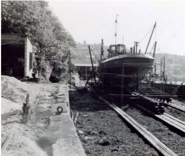
An early picture of the first tug Cannis on the slipway showing the restricted access between No 1 and No 2 slipways and the access to the port side of the ship for working
