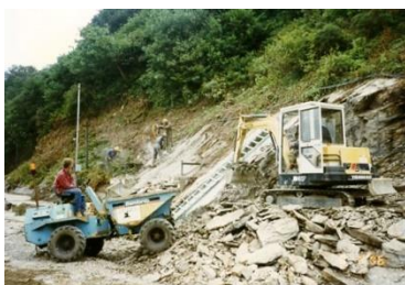
The removal of rock and fill more blasts to bring down the cliff in controlled explosions
