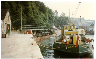
Lantic Bay bringing in sand and shingle infill with the sea wall at half height
