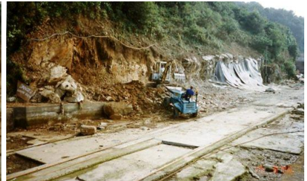
Rubble from the winch house and first rock fall taking the cliff away and loading a dumper For fill for the jubilee infill
