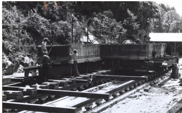
Polperro storm gates on the No 1 slipway cradle
