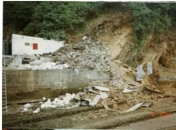
Rubble from the winch house and first rock fall taking the cliff away and loading a dumper For fill for the jubilee infill
