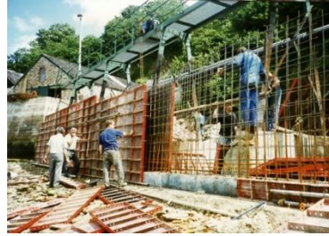
Concrete was pumped in from Toms Yard before raising the wall and commencing the infill
