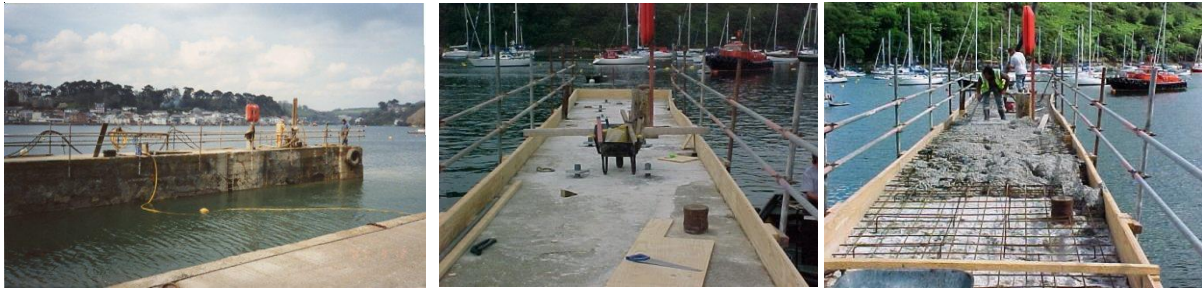
Drilling in tie rods before laying a new reinforced concrete top
