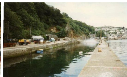
The removal of rock and fill more blasts to bring down the cliff in controlled explosions
