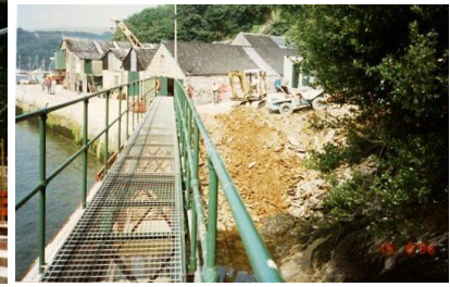
Concrete was pumped in from Toms Yard before raising the wall and commencing the infill
