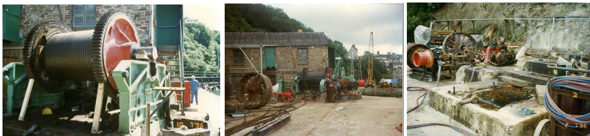
The large drum being jacked up from its supports and the hug belt wheel dismantled and finally of its base
