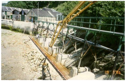
Concrete was pumped in from Toms Yard before raising the wall and commencing the infill
