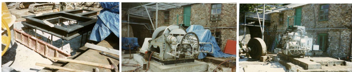
The base for the replacement Hydraulic winch. The winch motor in place
