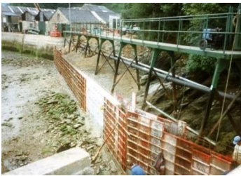
Lantic Bay bringing in sand and shingle infill with the sea wall at half height
