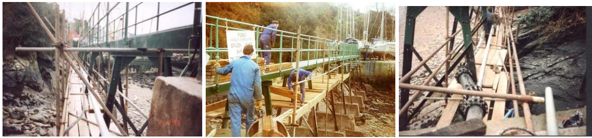
Preparing to run the sewage, water and electricity supplies under the bridge.
