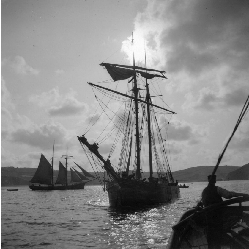
A picture from the tow deck of the Countess of Jersey
